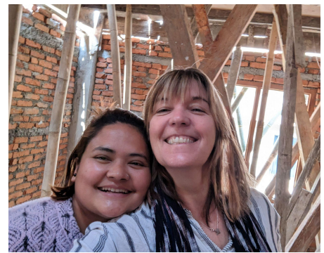
Anjali & Me in the dorms under construction
